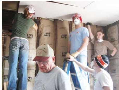
STA students installing drywall in a Cedar Rapids residence
